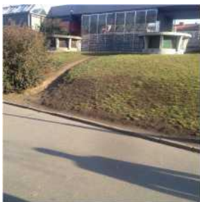
11. footpath leading to the problematic area next to the station hall
